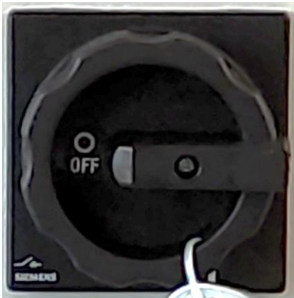
Figure 13: Main door switch – shown in "OFF" position (exact orientation of the switch may vary)
